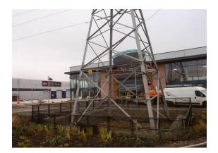
Externally there is perimeter fencing to the retaining wall to the rear of the service yard and to the base of the electricity pylon to the northern elevation. The car park is drained through two petrol interceptors. Two lagoons have been created to control the surface water to the west of the site. The rainwater from the building feeds into the underground attenuation system.
